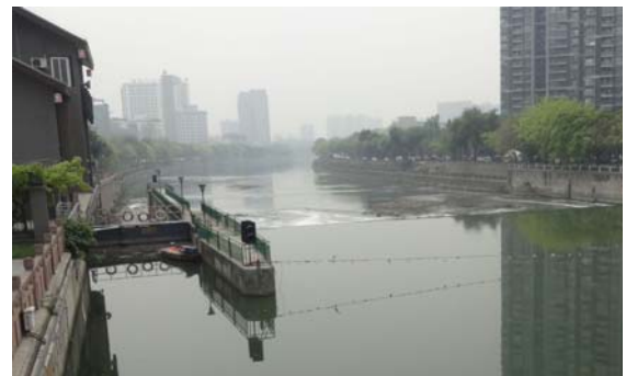
Funan river lock and dam
