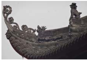
A typical roof corner
