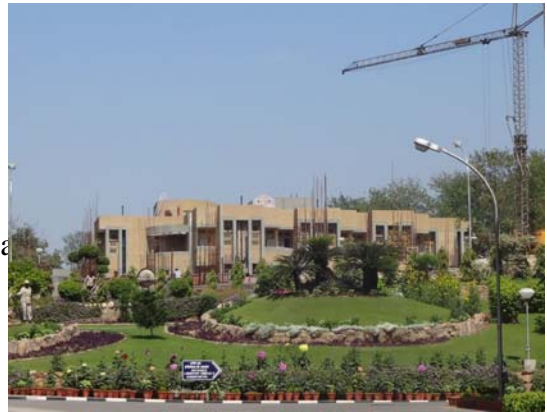
Overview: construction site is between grassy knole and the residence hall.
