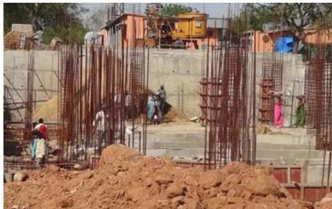
Working in the construction site
